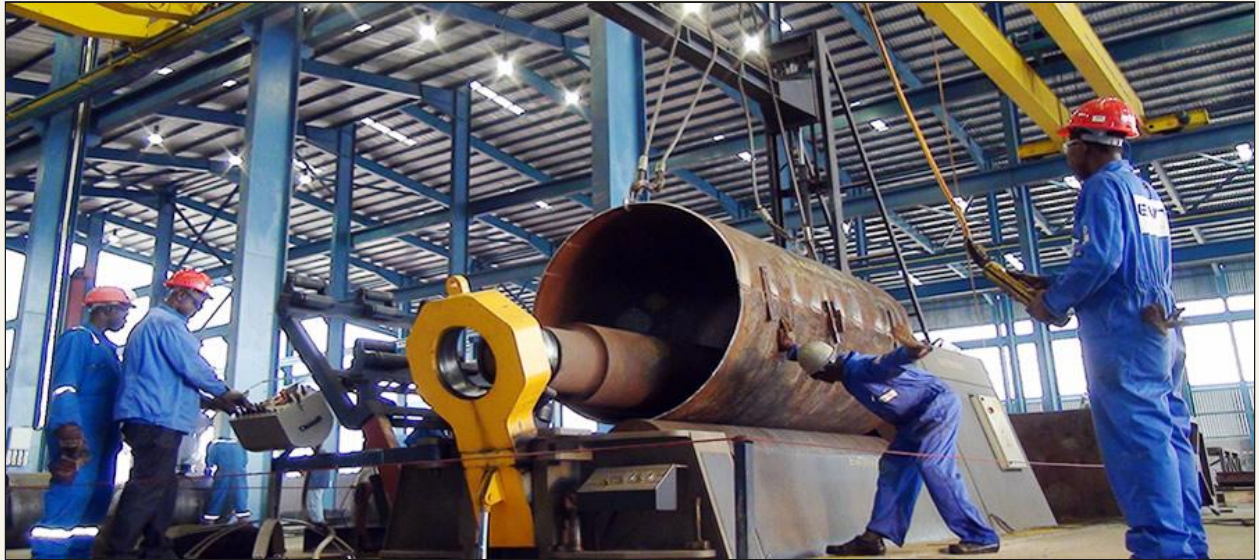
Nestoil Industrial Area — Building Indigenous EPC Capacity.
