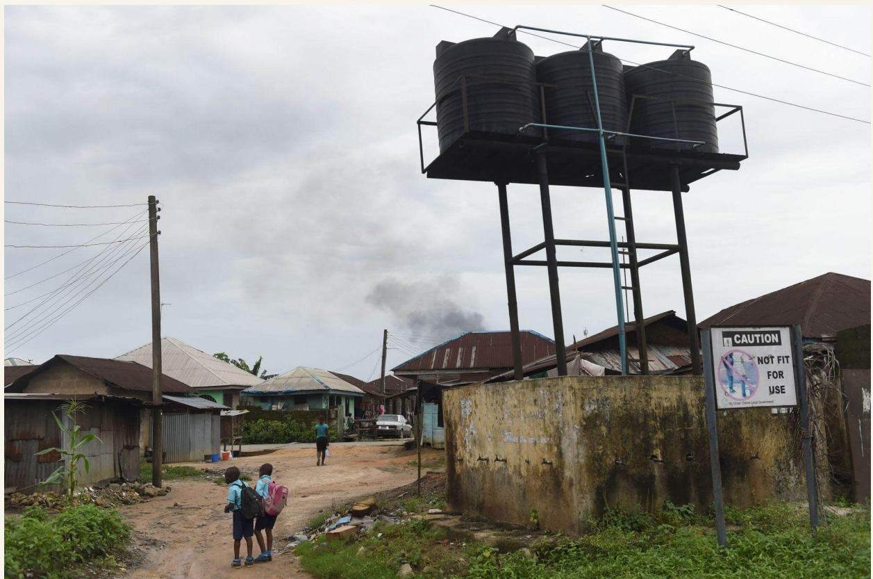
Water storage infrastructure bearing a caution notice. A facility is not a solution merely because it has been built.
