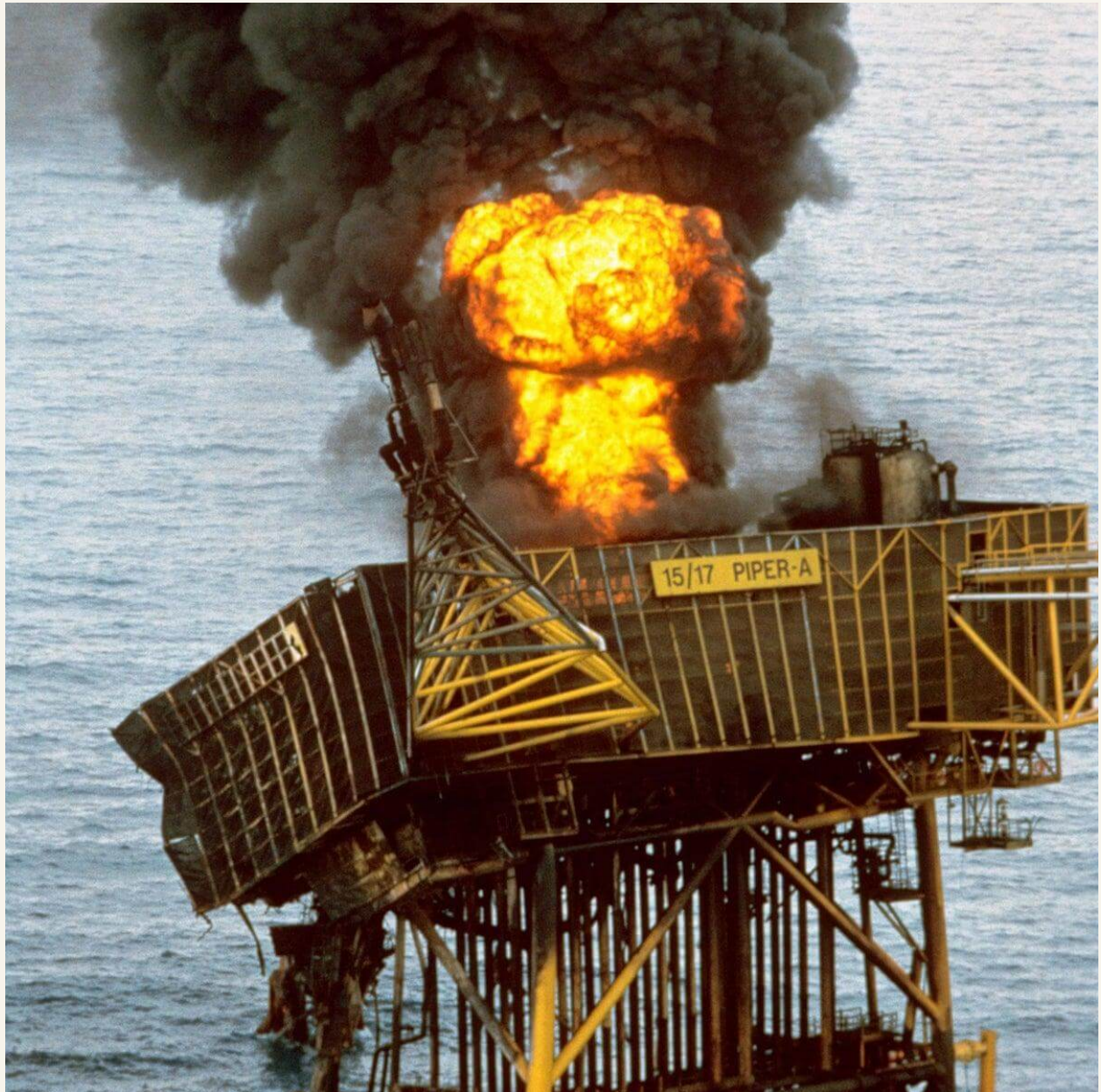
The night Piper Alpha burned: fire and smoke during the disaster.
