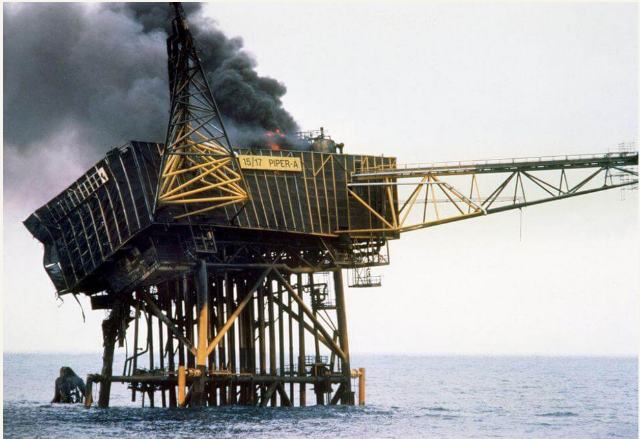
The aftermath that forced reform: the remains of Piper Alpha's A module the morning after the disaster.
