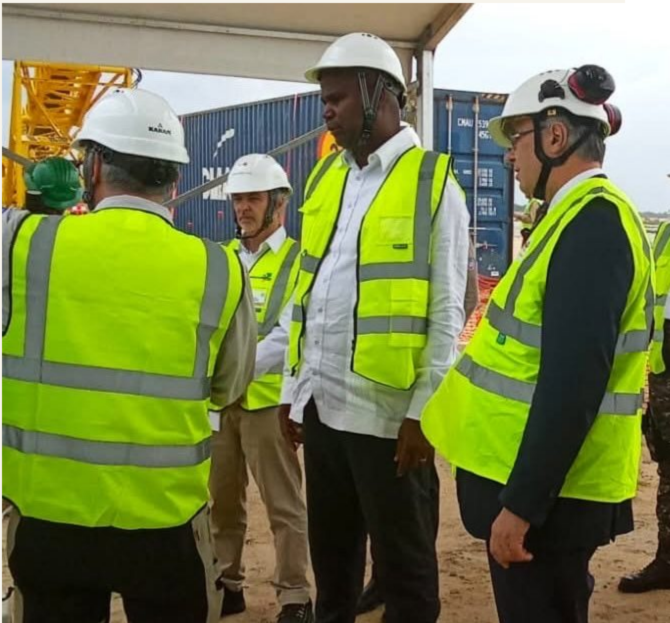
The Afungi Peninsula construction site, where work on Mozambique's $20 billion LNG project stood frozen for four years after the 2021 Palma attack.
